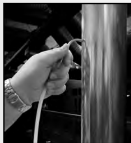
Place true draft hose and probe tip in flue to measure draft. You can also use the combustion draft probe for measuring pressure.
