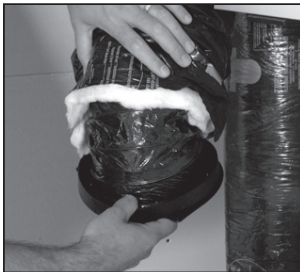
Figure 9 Insert flexible duct over the hooks and seal with a tie wrap.
