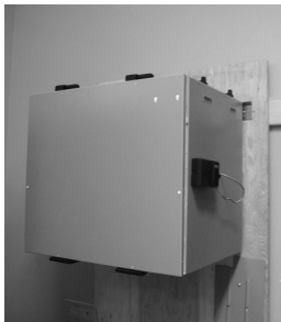
Figure 6 Hang HRV/ERV on the wall-mounting bracket.
