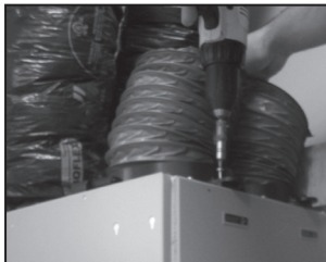
Figure 13 Fix and secure the collars to the HRV/ERV with the #10 x 1 1/4" screws, supplied in kit.
