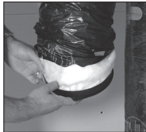
Figure 10 Insert insulation inside the double collar.
