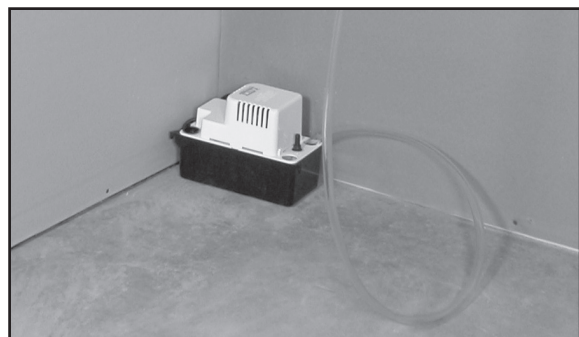
Figure 15 Use a condensate pump if you don't have access to a drain.
