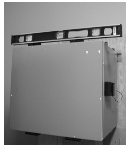
Figure 7 Before completing the installation, make sure that the HRV/ERV is level.
