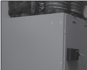
Figure 12 Slide collar into the keeper section of the unit.
