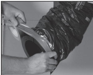
Figure 11 Finish by taping the vapor barrier to the collar to ensure proper seal.
