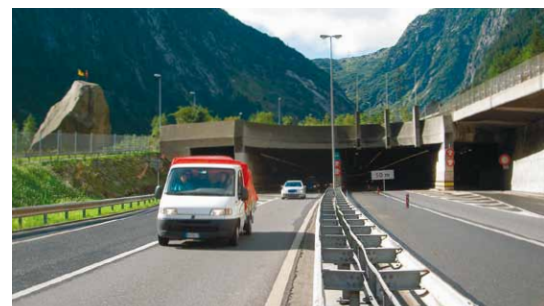
CLIC has proved itself in numerous road tunnels such as the Gotthard tunnel in Switzerland.
