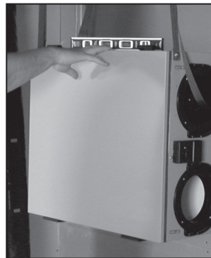
Figure 6 When the HRV/ERV is hung, ensure that the HRV or ERV is installed level for proper operation.
