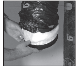
Figure 8 Insert insulation inside the duct and seal with the double collar.
