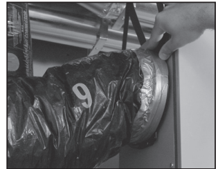
Figure 10 Slide collar into the keeper section of the unit.
