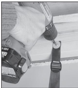
Figure 5 Attach the adjustable hanging straps to the floor joist with four, #10x1" screws. The screws are inserted through one of the links in the hanging chains.
