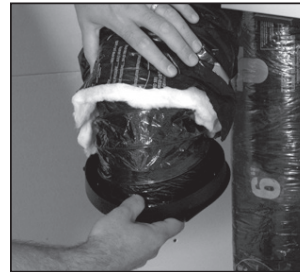
Figure 7 Insert flexible duct over the hooks and seal with a tie wrap.
