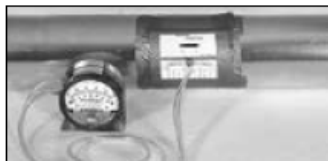
Seal airflow grid in duct with duct tape
