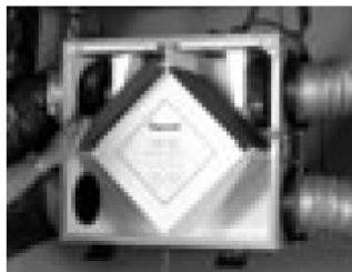
1. Slide out the filters.
