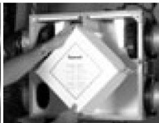
2. Slide out the energy core.
