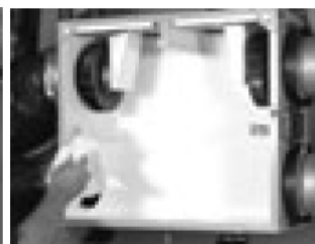
4. Wash out the walls of the unit.
