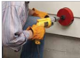
Cleanly cut holes in walls clad with FIBER CEMENT SIDING!
