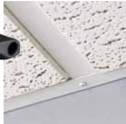
Work overhead and in tight corners!
