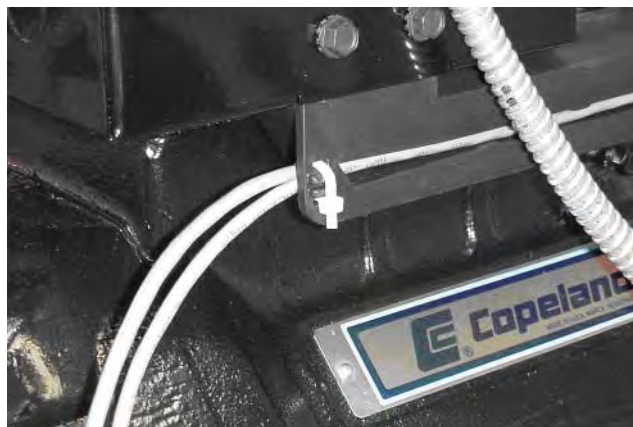
Figure 2.9 2D / 3D Communication Wire Routing
