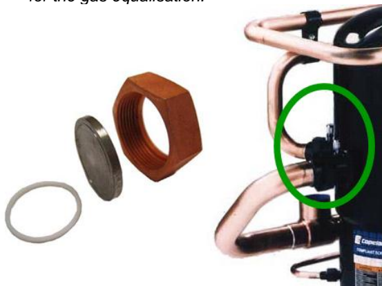
Figure 3: Blanking cap – gas equalisation
