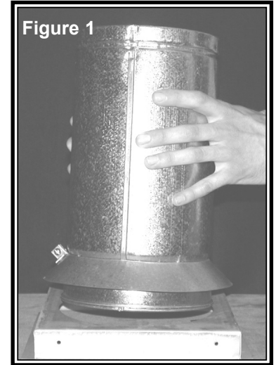
Figure 1 shows the installation of an RSA support assembly.
